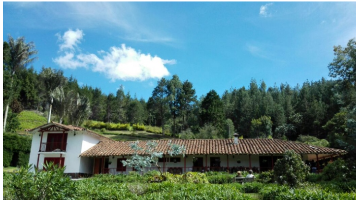
Vista General Centro Dhamma Gutti- Guarne Antioquia
